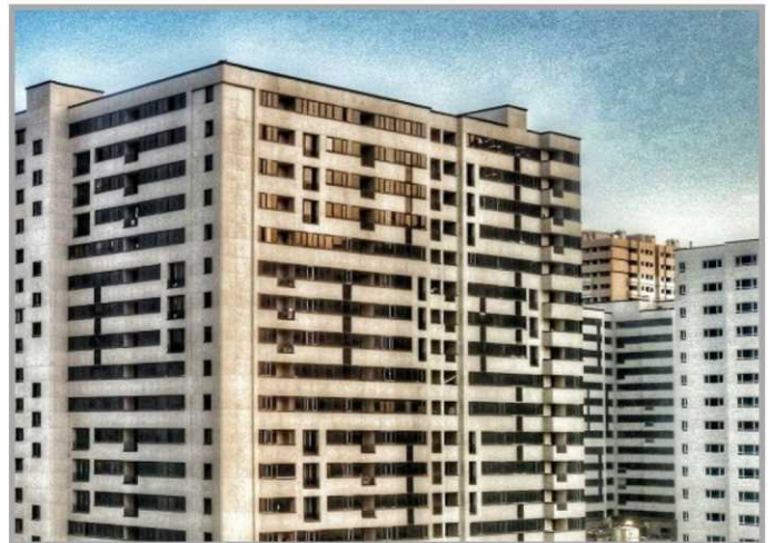
Ziton Tower (Tehran)
